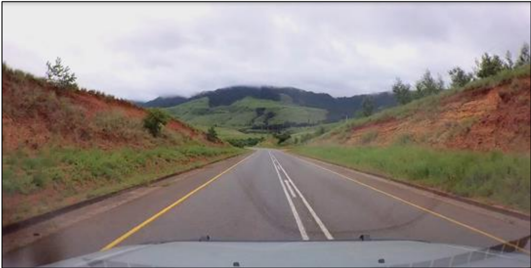
Figure 4-4: The existing Provincial Road R617 Cross Section through cutting
