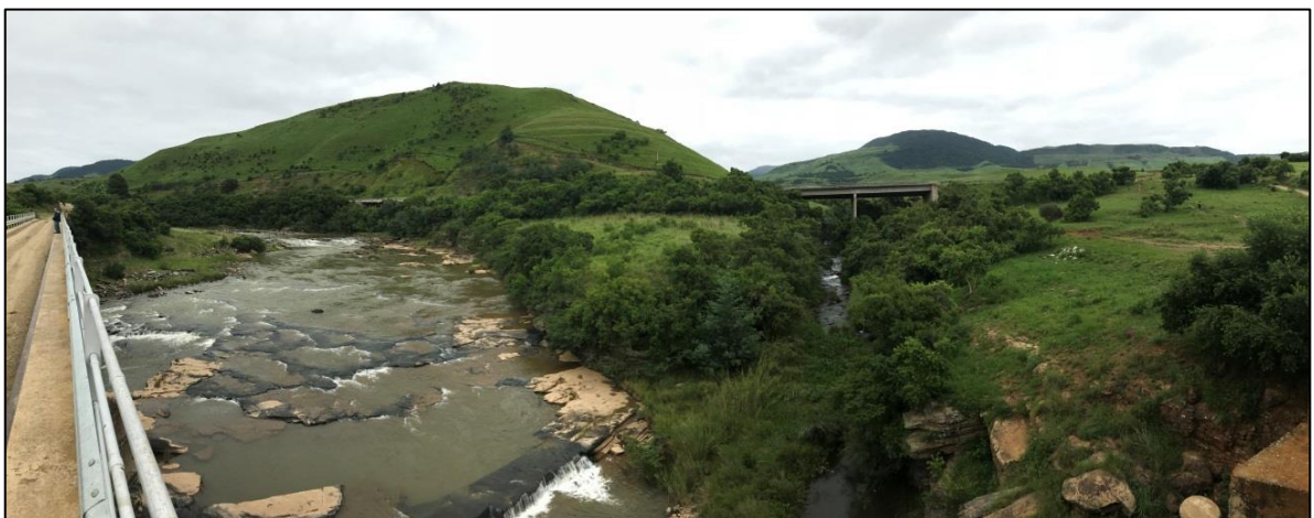
Figure 1-1: The old Deepdale Bridge on the left and existing the R617 Bridge to the right that will be inundated by the proposed Smithfield Dam
